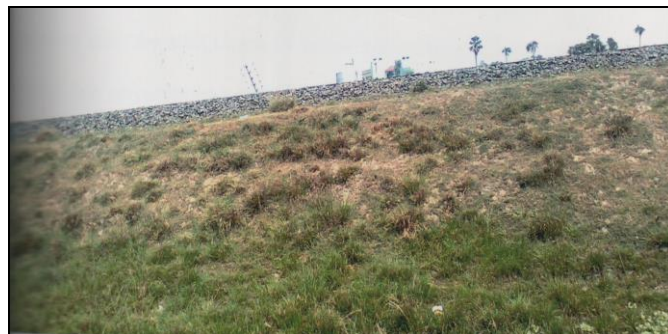
Fig 3: Vetiver hedges alongside a railway line
